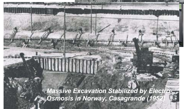
Electro-Osmosis Electrodes
