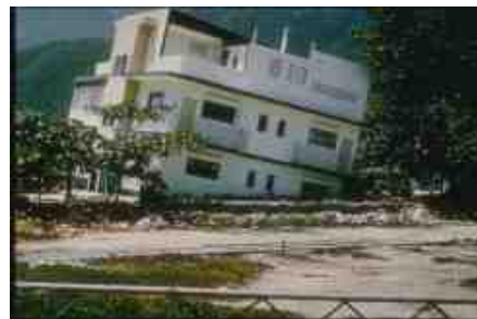
Buildings Destroyed due to Liquefaction of Subsurface Soils
