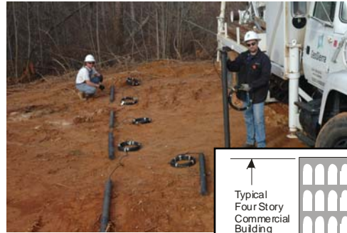
Electro-Osmosis Graphite Electrodes for GeoSierra's Quake Defense System
