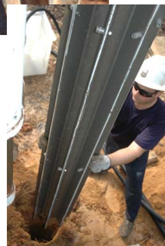
Each individual Frac Initiated & Propagated by Dedicated Tubing to Dilating Cavities in Production Version of STAR Frac Casing
