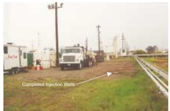
Above ground view of completed injected Reactive Barrier
