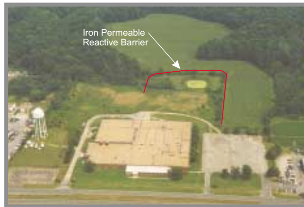
Aerial View of Iron Permeable Reactive Barrier
