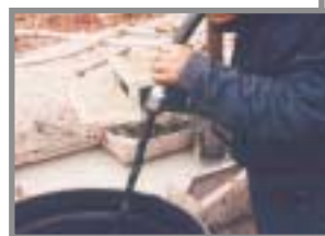
Injected Iron Slurry Mixture for Reactive Barrier
