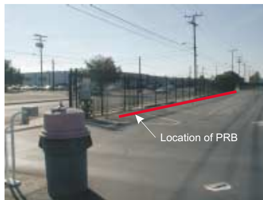
Location of Iron Permeable Reactive Barrier
