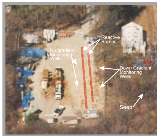
Aerial View of Reactive Barrier
