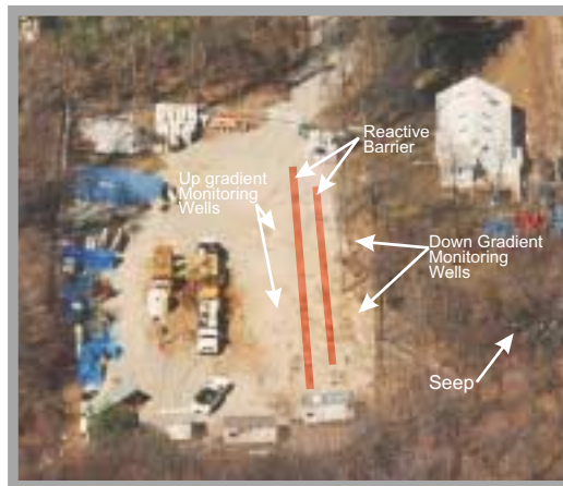
Aerial View of Reactive Barrier
