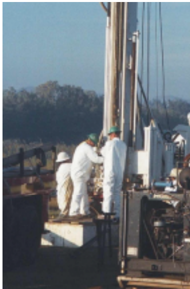
Installation of new azimuth control frac initiation casing system.
