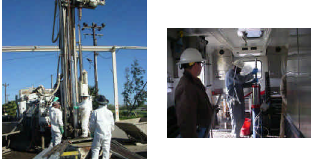
Figure 2. Hydrofracture Well Casing and Resistivity String Installation
