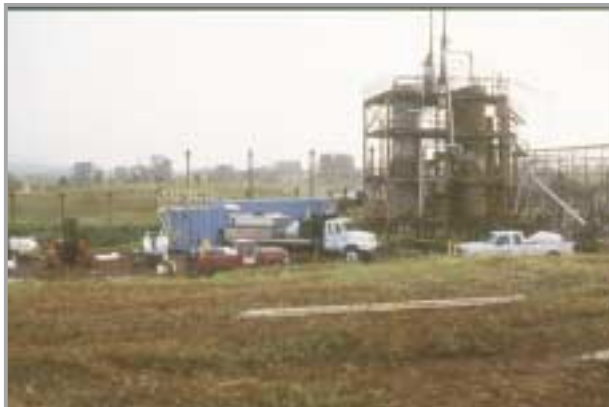
Groundwater Remediation at a TNT Manufacturing Facility using Hydraulic Fracturing
