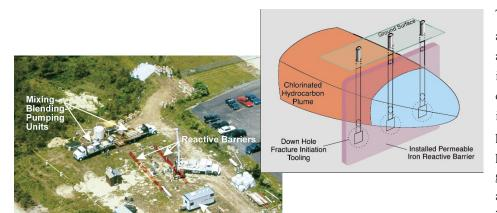
The in situ reactive barriers are constructed from a series of wells installed along the barrier alignment. A controlled vertical fracture is initiated in each well at the required azimuth orientation and depth. Iron filings are injected into the wells in a highly viscous cross linked proprietary HPG gel, to form a continuous permeable iron reactive barrier. The barrier's geometry is monitored in real time by the active resistivity method to ensure the barrier is constructed as designed.
